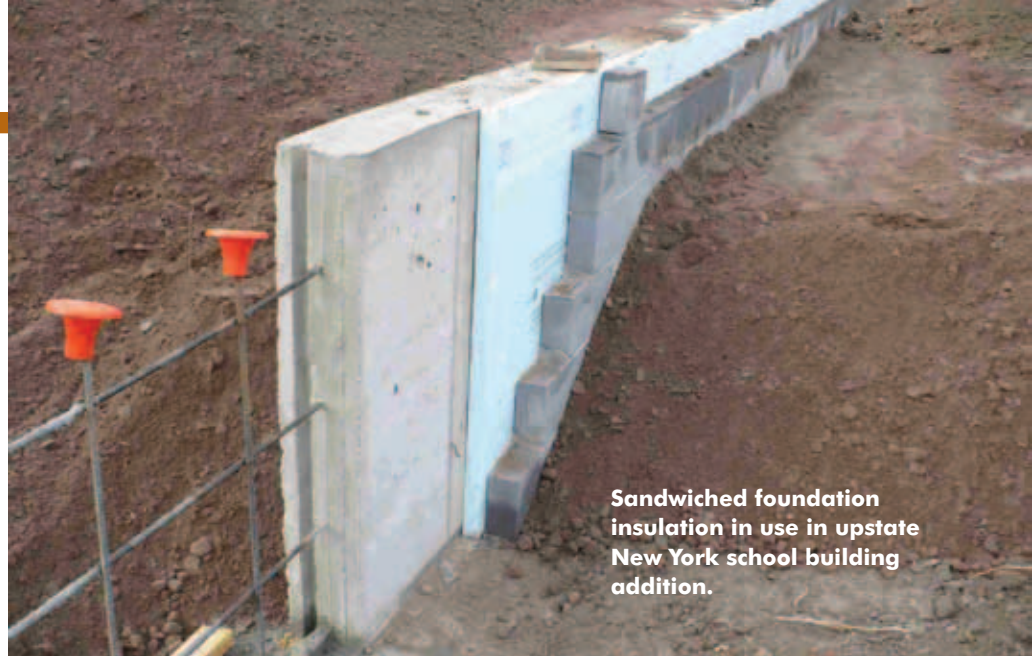
Foundation insulation on the outside face, inside face, and sandwiched inside.
